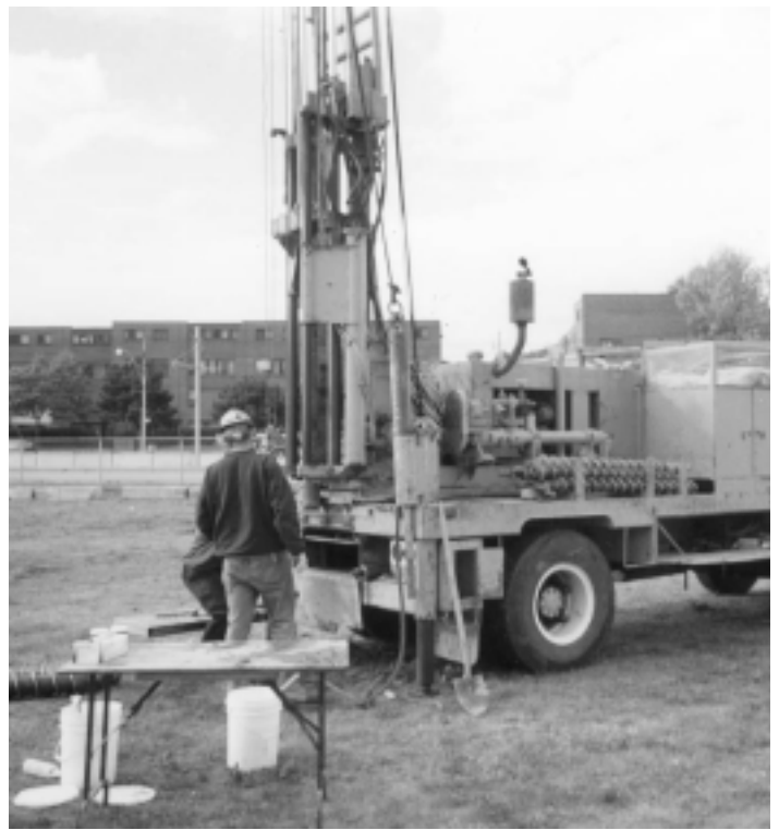
Drilling for soil and ground water analysis on the site
