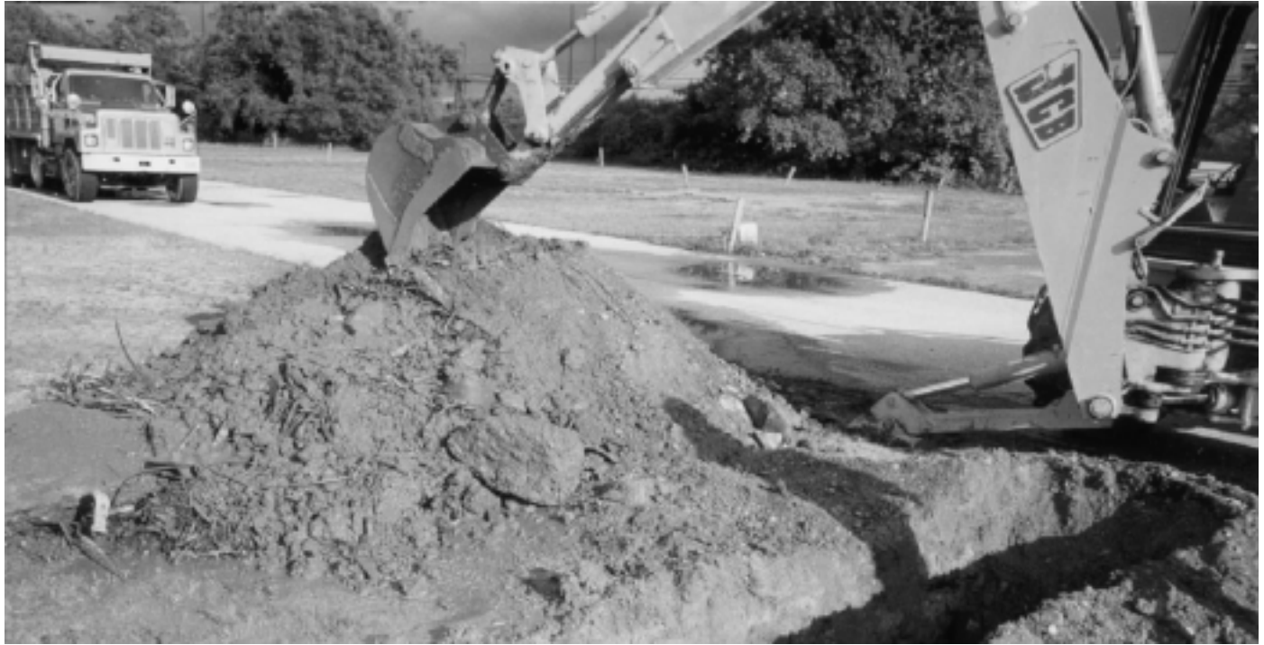
Careful soil excavation for testing and sorting
